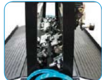
ADDITIONAL VALVE STORAGE IS LOCATED BETWEEN THE PANELS
